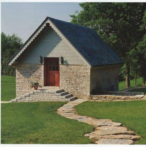
When updating the spring house on this historic property, the footprint of the existing masonry wall around the back of the structure was used as a strict guideline. Two of the original rooms can still be found beneath the main level; one that collected and pumped water and another that kept dairy products cool during hot summer months. Photography by Walt Roycraft.
